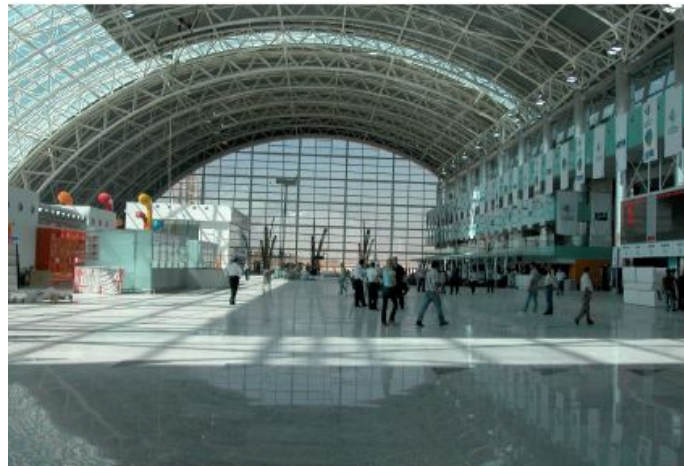
Figure 2 – ADB, Interior View (Ege Mimarlık, 2007).
